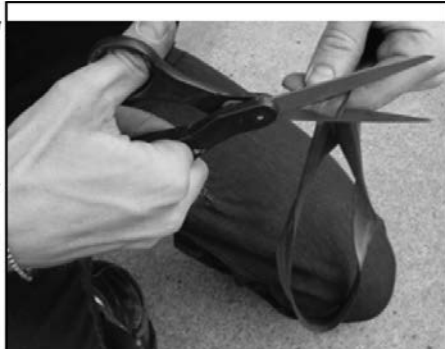
Cut hole for valve stem
